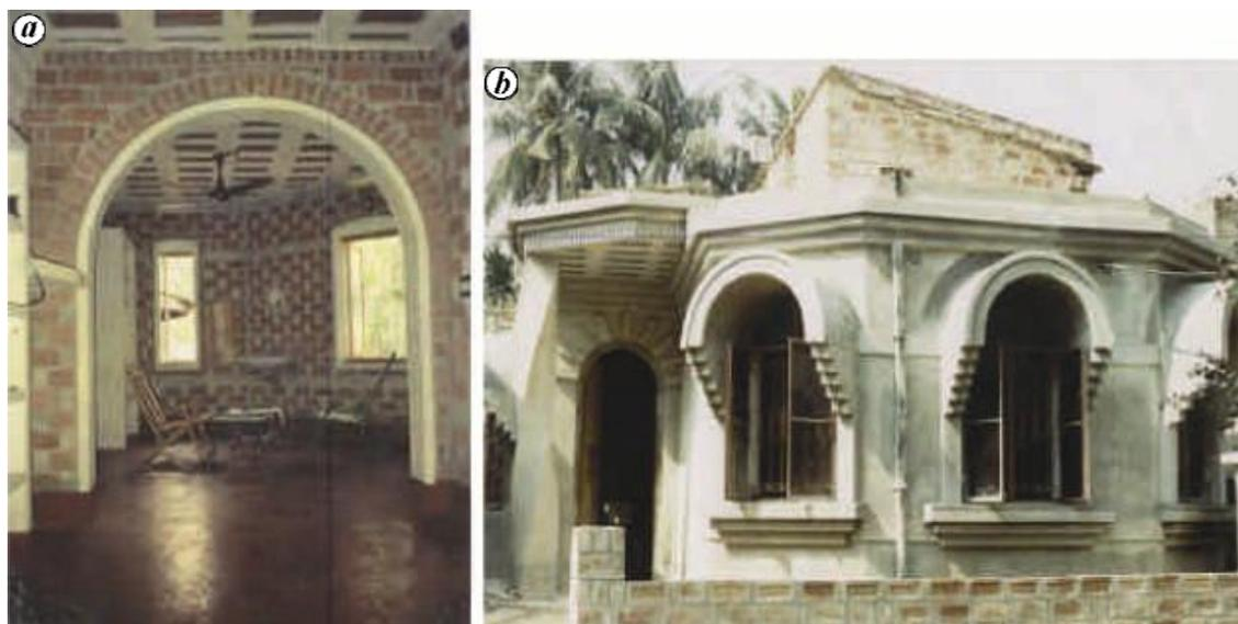
Figure 3. (a) Brick arch and (b) Brick corbelling (source: FOSET).
