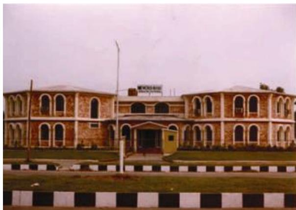
**Figure 6.** Office building with rat-trap bond wall, filler slab (source: FOSET).
