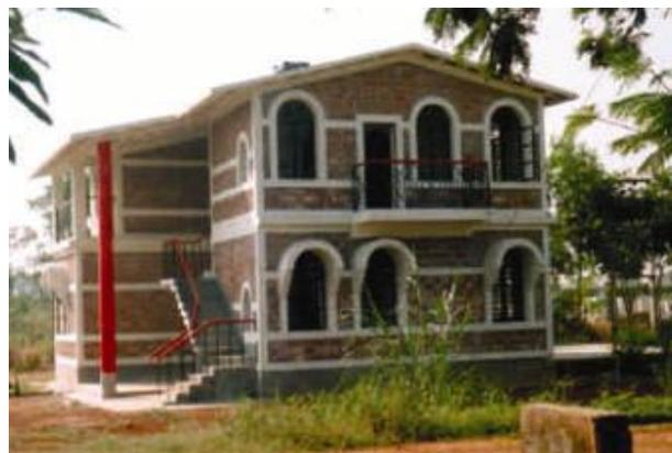
**Figure 2.** Two-storied building with rat-trap bond wall (source: FOSET).
