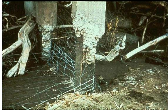
Fig. 1 Bridge Column in Sulphate Soils Due to External Sulphate attack.
