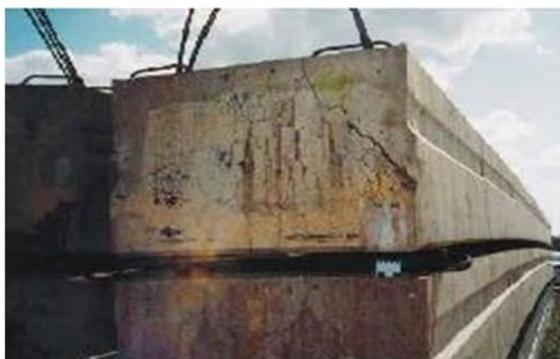
Fig.5. Spalling due to Sulphate attack
