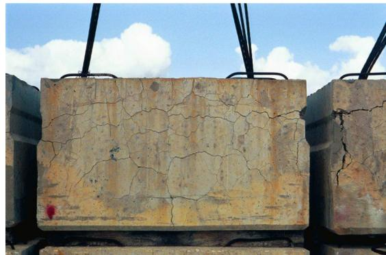
Fig.2 Concrete Box Beam due to sulphate attack
